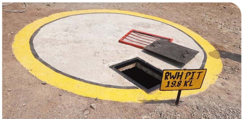
▲ Vyshali Energy Pvt. Ltd, Karnataka
